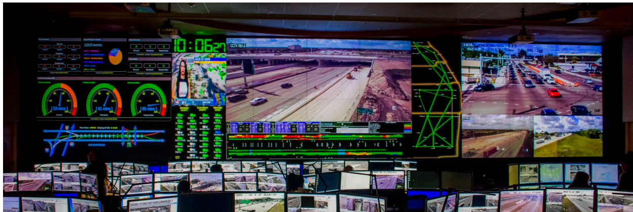
Figure 8: Florida DOT, District Four TMC Video Wall (Performance Measures)
