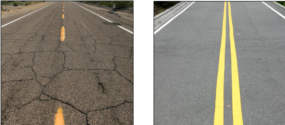
Figure 11. Photos. A severely cracked compared to a smooth pavement.
