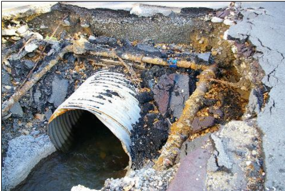
Figure 21. Photo. A deteriorated culvert.
