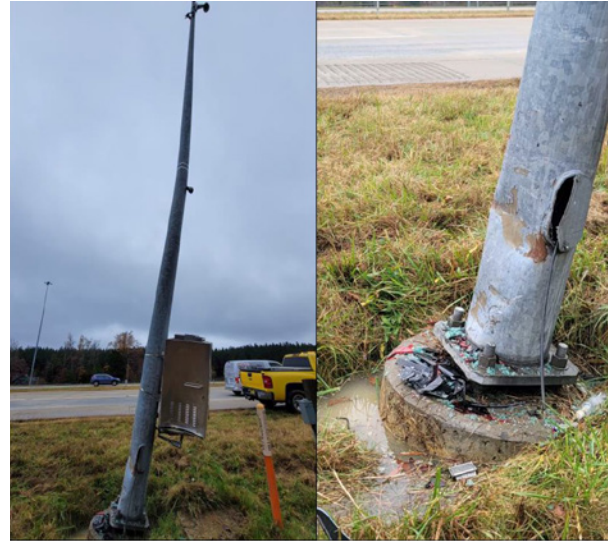
Damaged pole replaced utilizing responsive maintenance
