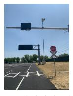
The assets designed and constructed include one ground mounted dynamic message sign and one cantilever dynamic message sign with their corresponding controller cabinets, lane use control signs (LUCS) that are being
