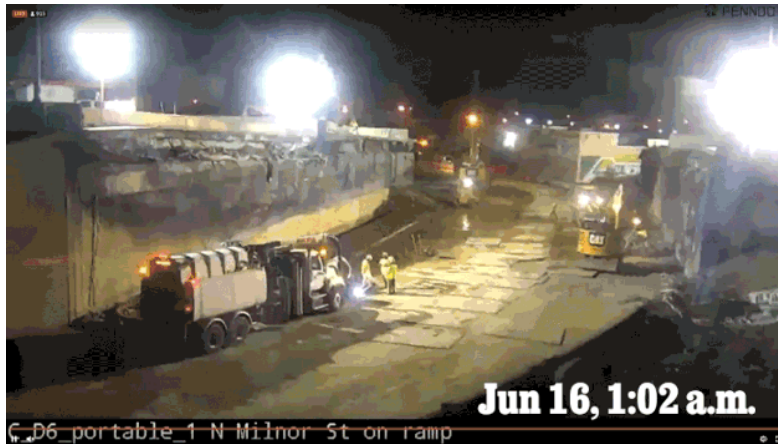
Figure 1: Live Stream Feed of I-95 Bridge Repair by PennDOT
