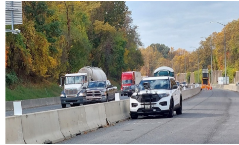
Source: Maryland State Highway Administration
